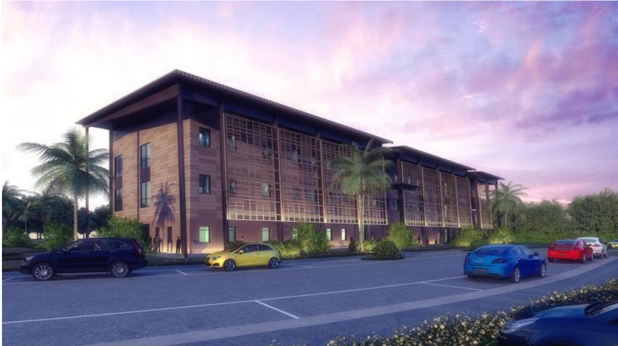
The DLR Group utilized a "modern agrarian" style for the new Poinciana Campus building, shown here in the southwest view. The metal grids on the side of the building are designed to provide shade, improve energy efficiency and protect migratory birds. (Valencia College)
